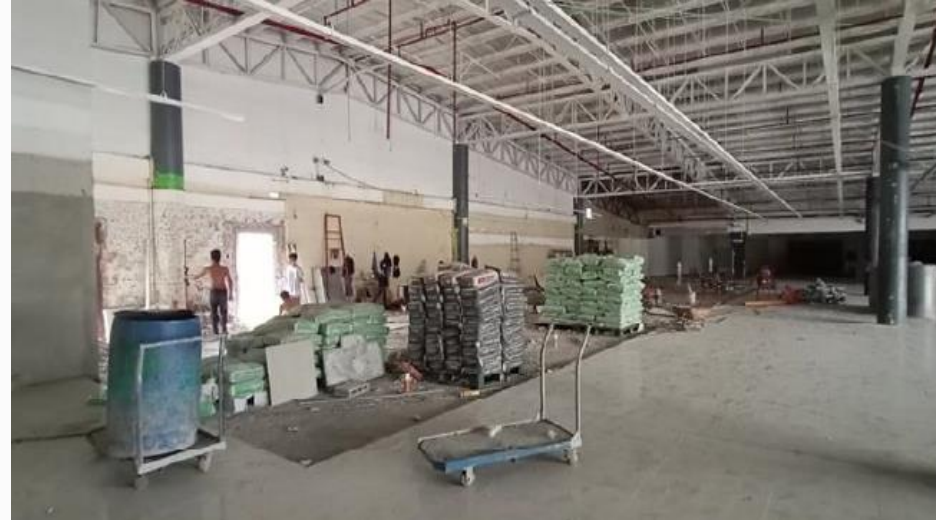
Fresh prep area and cold room
