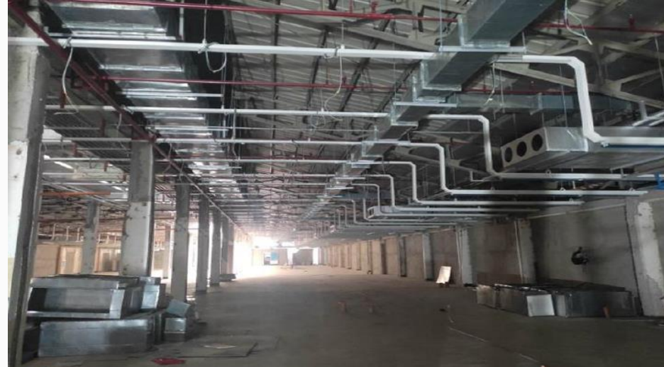
Selling area to supermarket entrance
